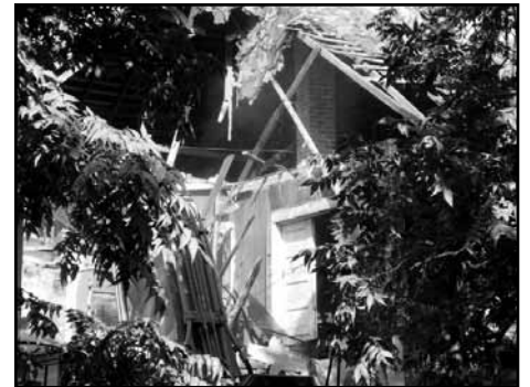
1900 5th Ave. — Demolition 2009.
