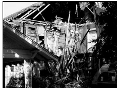
1900 5th Ave. — Demolition 2009.
