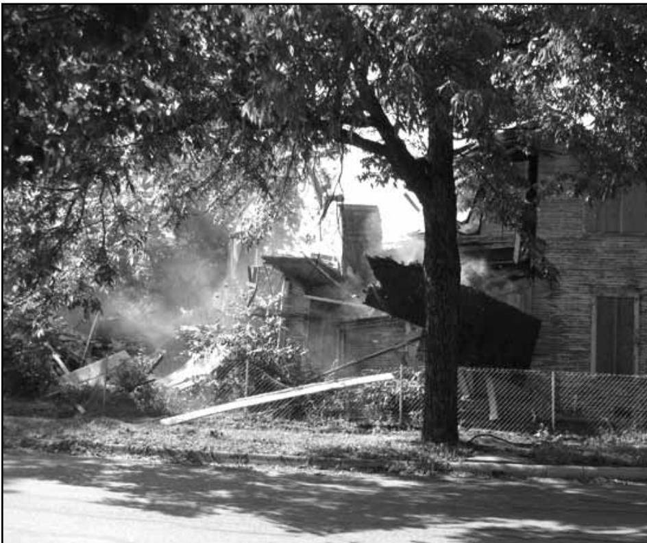
1900 5th Ave. — Demolition 2009.
