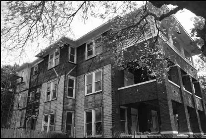
1507 Alston — bought and sold after three prior attempts to restore, the Bomar Building is very close to being finished as six completely renovated apartments with all wood restored flooring and win-
