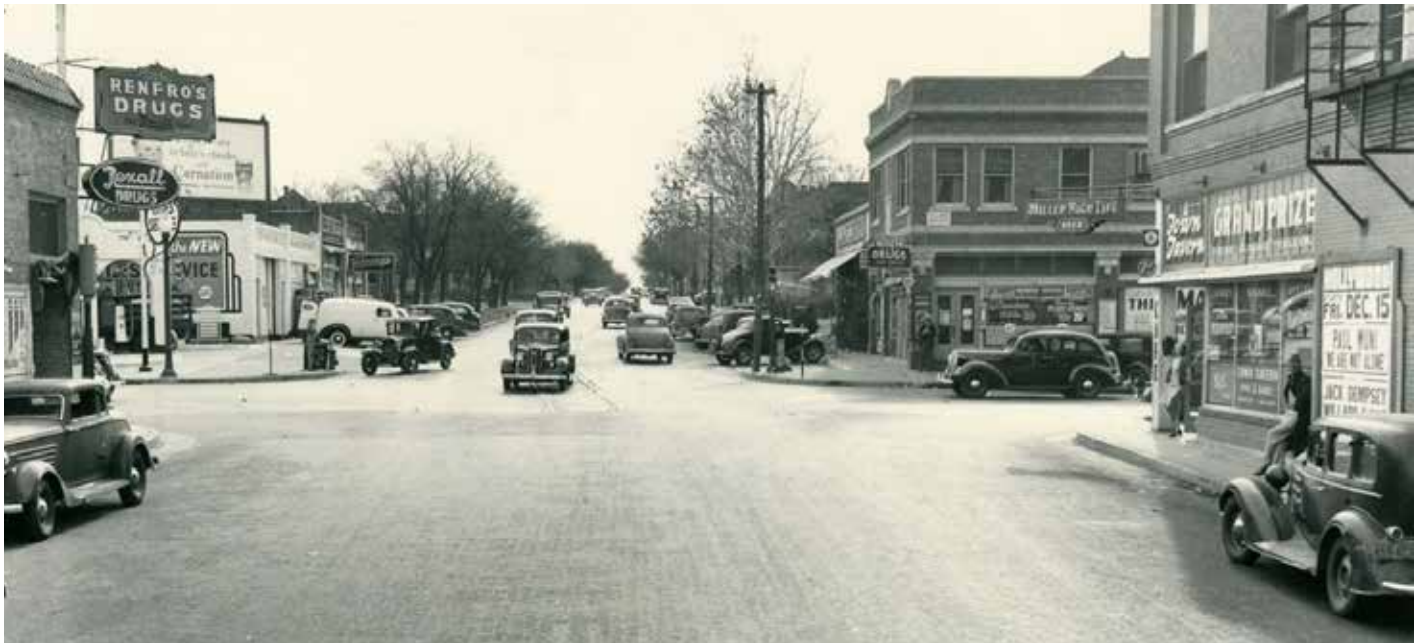
Photo courtesy Fort Worth South, Inc.
