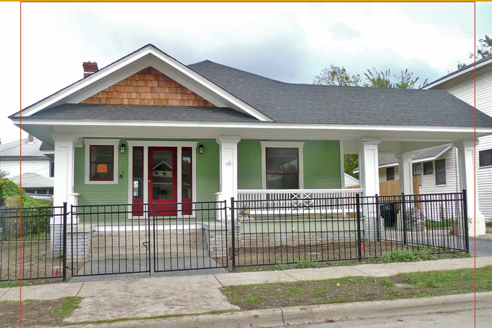
1405 Fairmount Ave. following renovation by owners Brian and Sheila Portwood. The house was scheduled for demolition in 2010.
