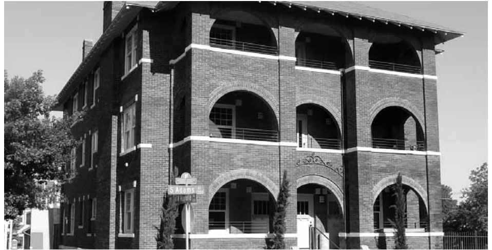
1228 South Adams St. — Excellence in restoration and adaptive reuse of a historic building.
