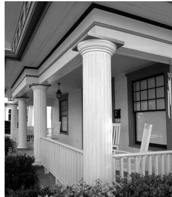
Large fluted Doric columns support an early enclosed sleeping porch on this 6th Avenue four-square. The 1x2 railing is very appropriate for the style.
