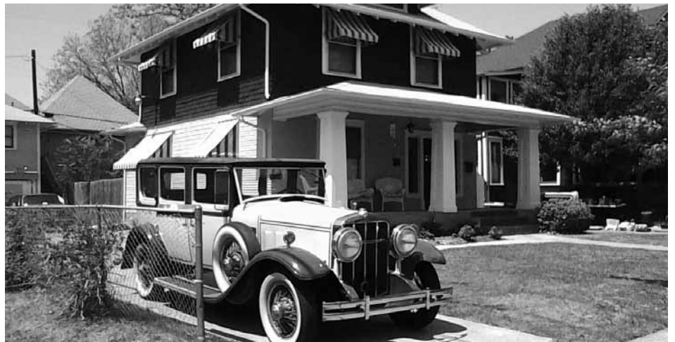
1912 Alston — Residential rehabilitation.
