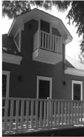
Deck—Railing--Balcony Rear Dormer
