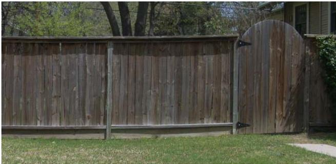
*LEFT: It is preferable for wood privacy fences to be capped. The wood cap helps to shed water, increasing the longevity of the fence.*
