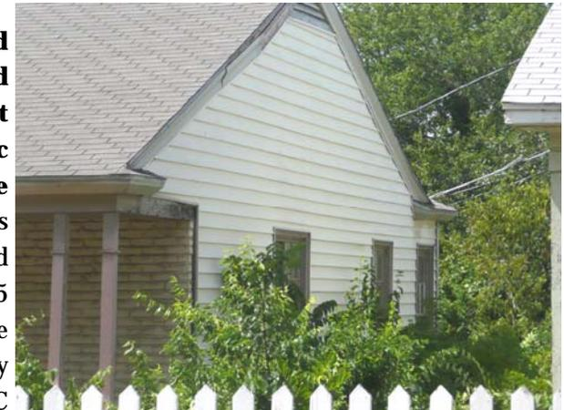
*ABOVE: The structure has a brick veneer on the front and inappropriate vinyl siding at the side.*
