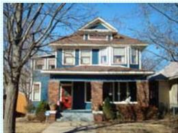
**Boxed Eave (boxed cornice):** A hollow eave enclosed by the roofing, the soffit, and the building wall.
